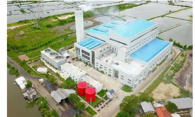
Benowo – Steam Gasification Producing electricity by Steam Turbine
